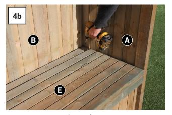
Position the Seas Hinged Assembly E on to the seat support battens (Fig.4a) and fix to the seat support battens using 4 x 60mm Screws – 2 per side of rear section of the Hinged Seat Assembly E (Fig.4b).
