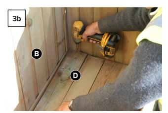
Locate Floor Panel D on to the floor support battens (Fig.3a) and fix to the floor battens using 4 x 60mm Screws - 2 per side.
