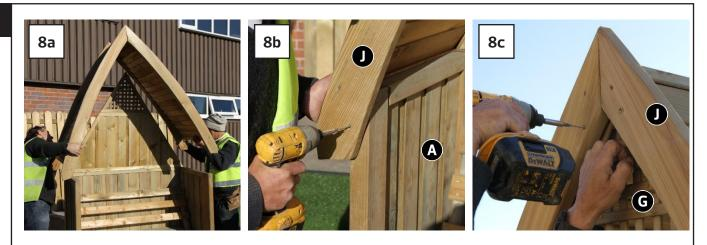
Place roof assembly on to Side Panels A (Fig.8a) and fix to the Side Panels A through Fascia Boards Jusing 4 x 60mm Screws – 1per Fascia Board. Further attach the roof assembly to the Trellis Back Panel G through the Fascia Boards Jusing 2 x 50mm Screws – 1no per rear Fascia Board J.
