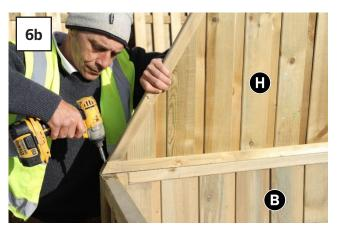
Attach Trellis Back Panel G to the Middle Back Panel H using 2 x 40mm Screws – 1 per side (Fig. 6a). Attach trellis and middle back panel assembly to the Back Panel B using 3 x 40mm Screws 1 per corner and 1 in the middle (Fig.6b).
