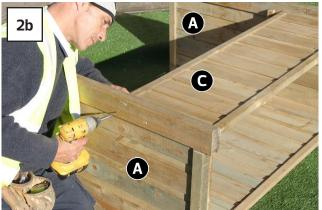
Place Front Panel (C) between the Side Panels (A) (Fig.2a) and fix in position using  $4\times60$ mm Screws – 2 per side (Fig.2b).
