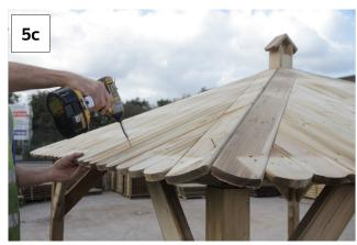
Locate Roof Panel G on to ring beam assembly and Roof Support F and fix in position using 6x 35mm screws (1 to Roof Support, 5 to ring beam).
