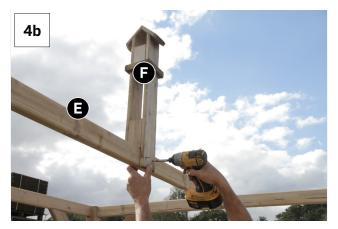
Fix Support Beam E centrally along ring beam assembly as shown in Fig. 4a using 4x 60mm screws. Position Roof Support F to the centre of Support Beam E and fix using 2x 35mm screws. (See Fig. 4b)
