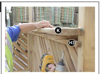
Position Back Shelf J and Side Shelves K onto shelf support battens and fix in position using 18x 60mm screws (6 per shelf). (See Fig. 7)
