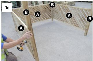
Attach Back Panel A to 2x Posts B at a nominal height of 150mm from base of posts, ensuring notches (cut outs) to posts are positioned externally and panel is flush with back of post using 6x 60mm screws (3 per post). (See Fig.1a) Attach Side Panels A to post/panel assembly using 6x 60mm screws (3 per post). (See Fig. 1b)
